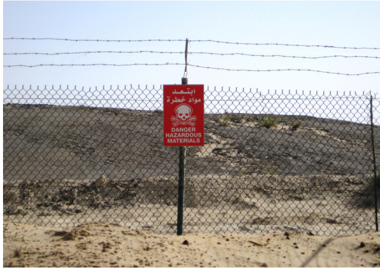
Figure 6-16 The Hazardous Waste Expansion Area (view to the northwest)
